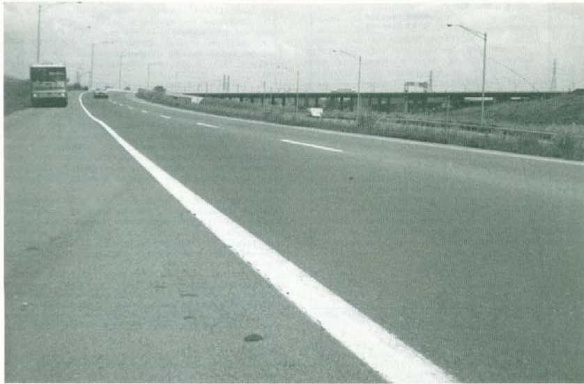
FIGURE B Interstate 85 westbound, 3 years after construction.
