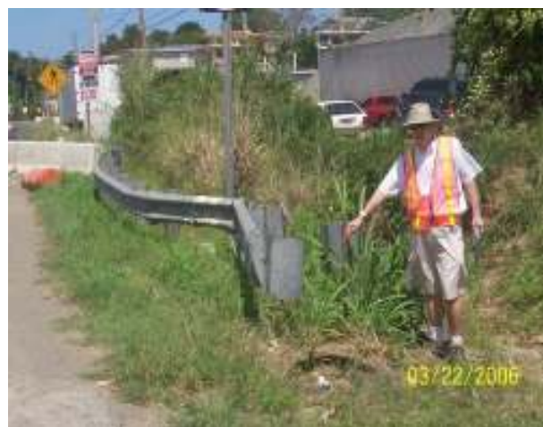
Unacceptable strong post block outs according to NCHRP 350
