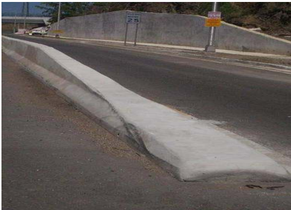
Inadequate color on the barrier and on the end treatment
