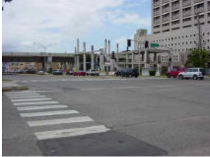
Fig. 13 Station construction view
