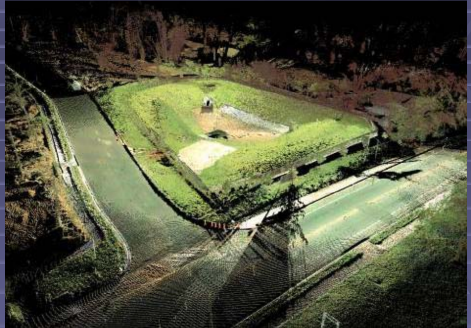
Holding Pond Survey
