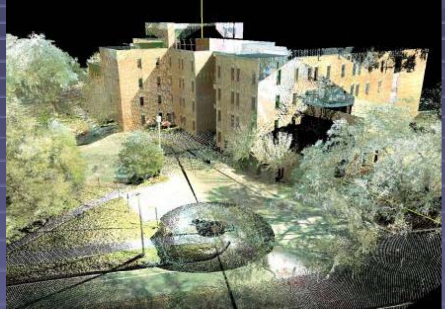
Stone Building @ FSU
