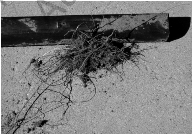
FIGURE 4 MRoots penetrating a drip emitter.
