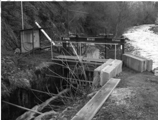
FIGURE 8 An example of irrigation district river diversion in Oregon [12].
