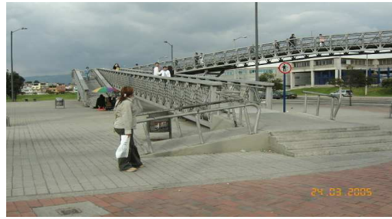
Access to a Pedestrian Bridge
