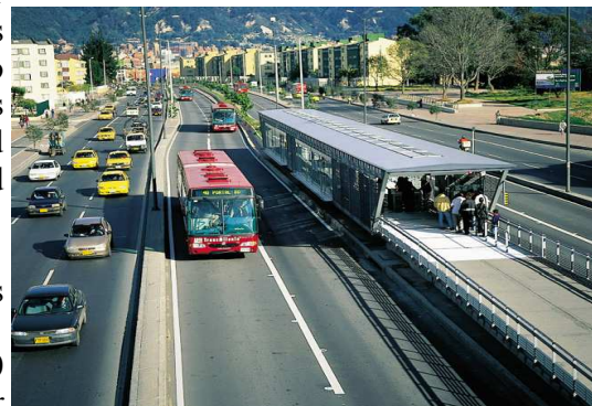
Exclusive Lanes and Simple Typical Station of a BRT
