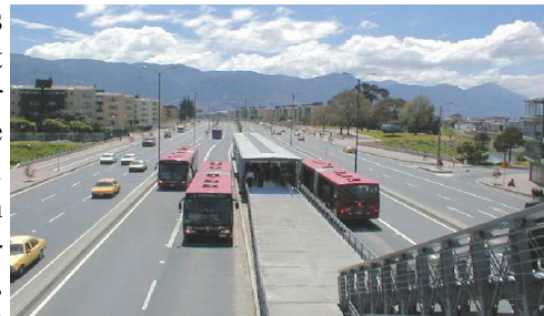
System Station with Articulated Buses
